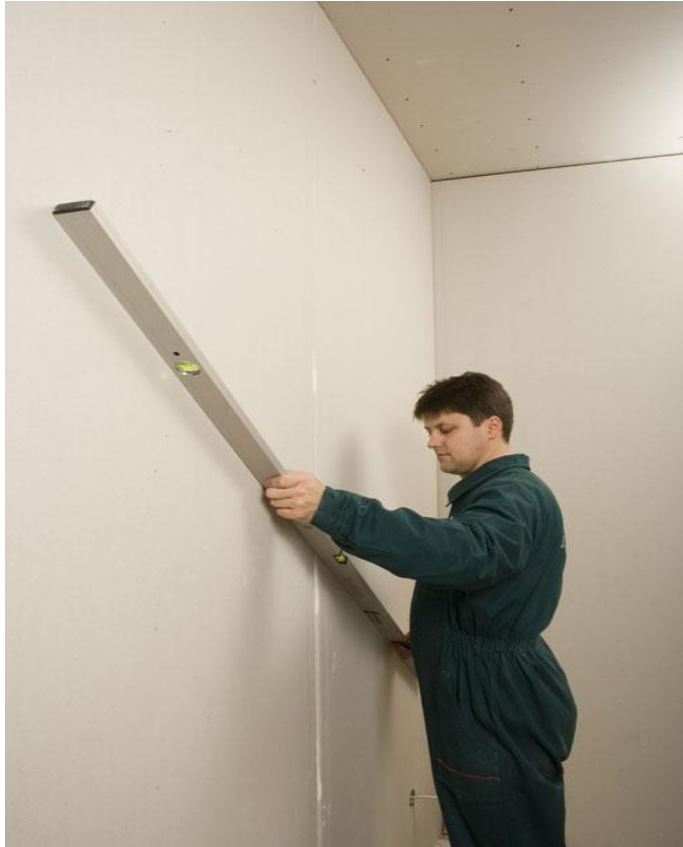
Fig. 4 Checking the surface and edge deviation from the vertical direction
