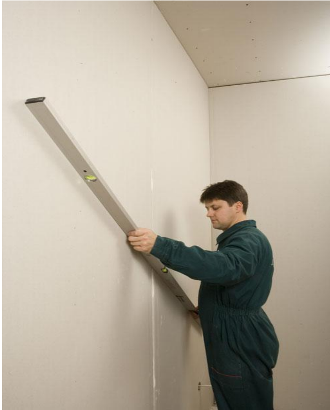
Fig. 11 Checking the surface and edge deviation from the vertical direction
