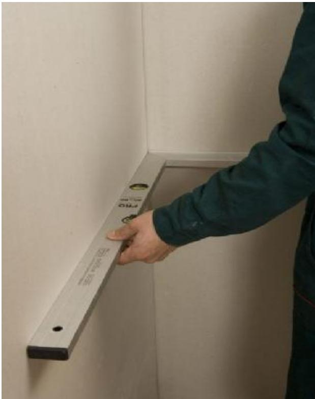
Fig 12. Checking deviation of intersecting planes from the angle specified in the documentation.
